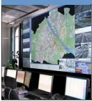
The traffic control computer supports the implementation of control, management and information strategies for traffic in Vienna. With this innovation, Siemens offers traffic-dependent management of traffic lights. Following the replacement of standard bulbs with LEDs from Osram, traffic lights consume 90 percent less electricity. The cost savings for the City of Vienna amount to around € 1.7m p.a.
