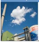
Steam generator with circulating fluidized bed firing and intermediate superheating. Intermediate fuel storage with conveyor system. Complete electrical and control-engineering equipment, including integration into the existing power station. In the new biomass power station 200,000 tons of wood trimmings and off cuts, bark and unpolluted old wood will be burnt. Reduction of CO2 emission by 144m tons p.a.
